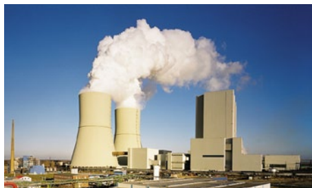
Different requirements of power plants require special gear unit solutions.
